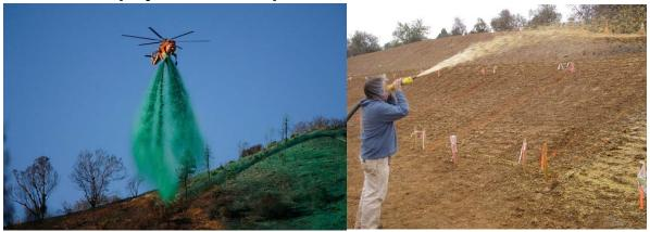
**What** – Combinations of organic fibers (e.g., wood shreds, paper, cotton, flax, etc.), tackifiers (i.e., glue), suspension agents, and seeds are mixed together with water and applied to the soil surface via ground or aerial applications.
