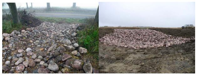
**What** – Structure made of rocks, logs, or plant material installed in ephemeral channels at the grade.
