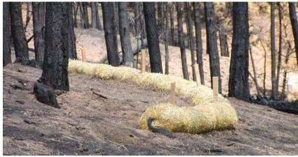
What – Fiber rolls, commonly called wattles, are prefabricated rolls manufactured from rice straw and wrapped in degradable netting. In some cases, on-site woody debris can be rolled in netting to reduce costs. Rolls are  $\sim$  9 inches in diameter and up to 25 feet long.
