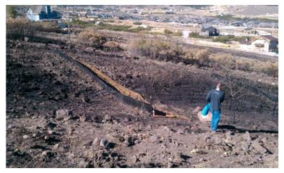
**What** – a permeable fabric installed parallel to the contour and anchored with wooden stakes or metal t-posts.
