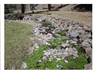
**What** – Reinforcement of streambank with protective covering, such as rocks, vegetation or engineering materials (including boulders, riprap, and gabion baskets).
